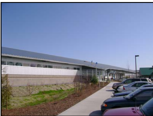
View of a portion of the industrial facility rooftop where the solar panels will be installed
